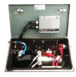
The **Safe-Away® 2009 Series VHS Power Pack** is driven by the Access Control System. The stainless steel VHS Power Pack cabinet houses the main control hydraulic and electrical components.
