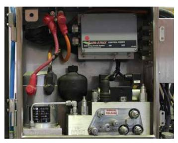
The **Safe-Away® 2009 Series Power Pack** is driven by the Access Control System. Conveniently, the top step/platform is the Power Pack box designed to safely store the hydraulic Safe-Away® Series 2009 Power Pack in a horizontal position. Or the Power Pack may be mounted vertically at another location of your choosing.
