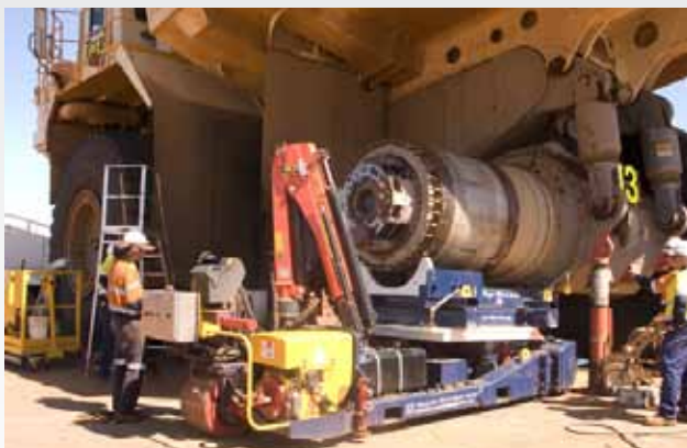
Terex MT6300 Wheel Motor removal using the Trilift® VWT XC30
