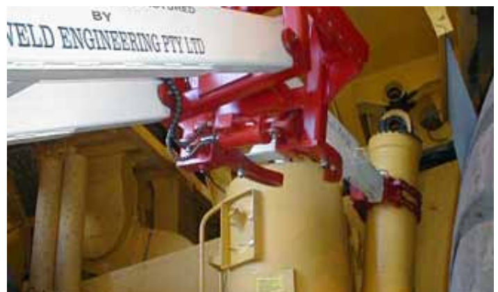
Hoist cylinder removal with VWT 15 and Multijig 15 with Universal Cylinder Clamp
